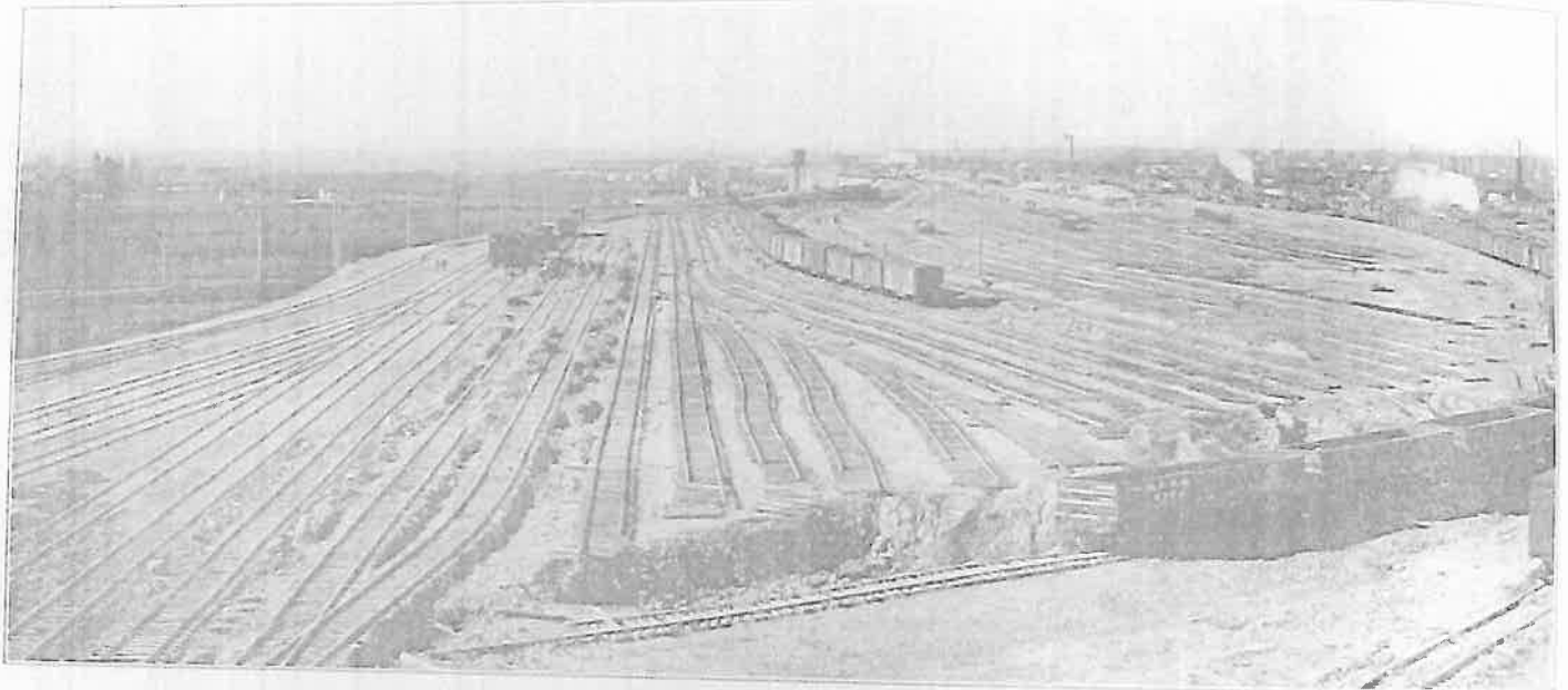
General View of Yard Under Construction, Looking West From the New Coaling Station
